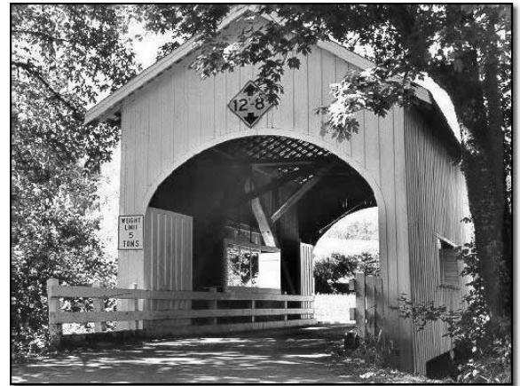
South Myrtle Creek (Neal Lane) Bridge (1939)
